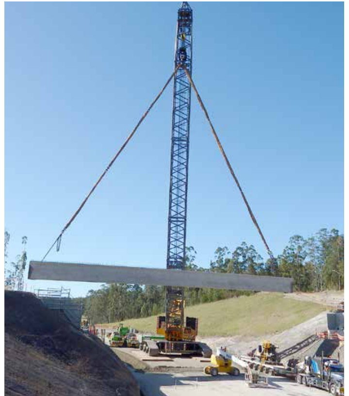
Lifting the single span girder onto Cockburns Lane bridge
